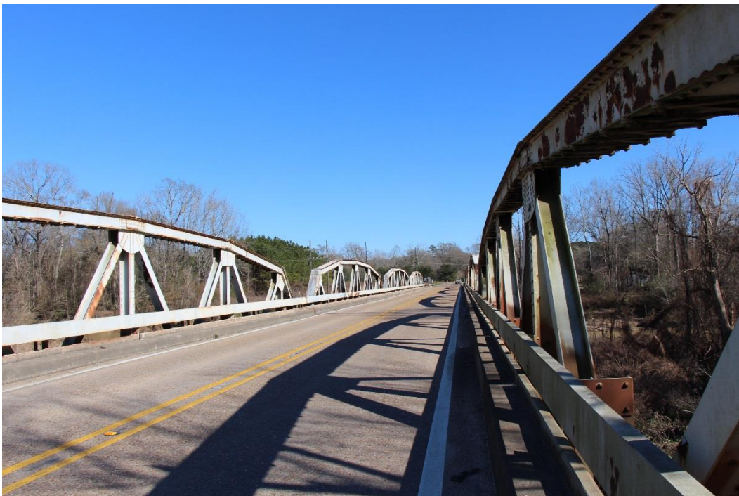
Historic Fabric Photo 3: Simple metal railing on the truss main spans.
