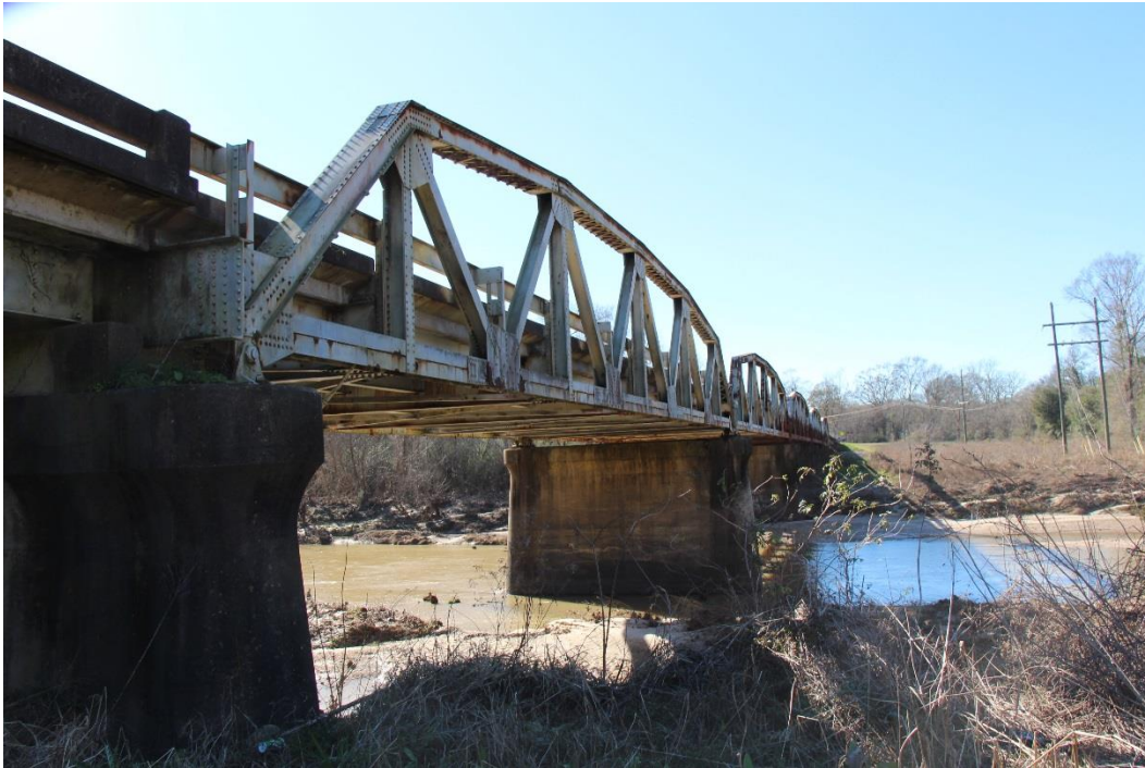
Historic Fabric Photo 2: Truss floor system and bridge substructure.
