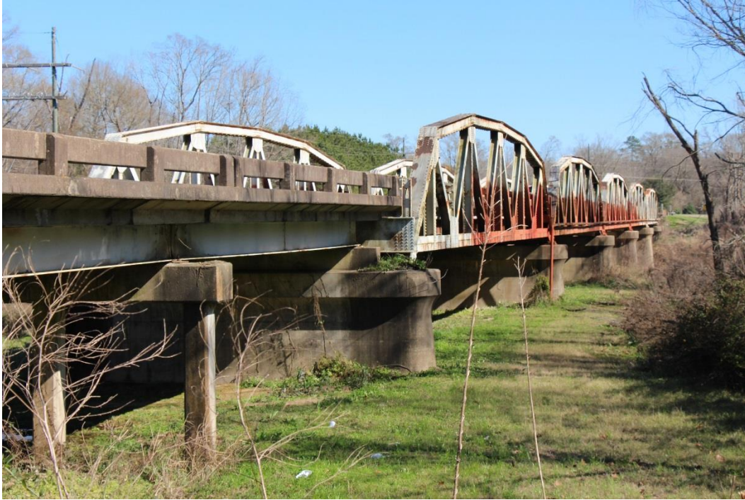
Condition Photo 3: Elevation view of the bridge, looking east.
