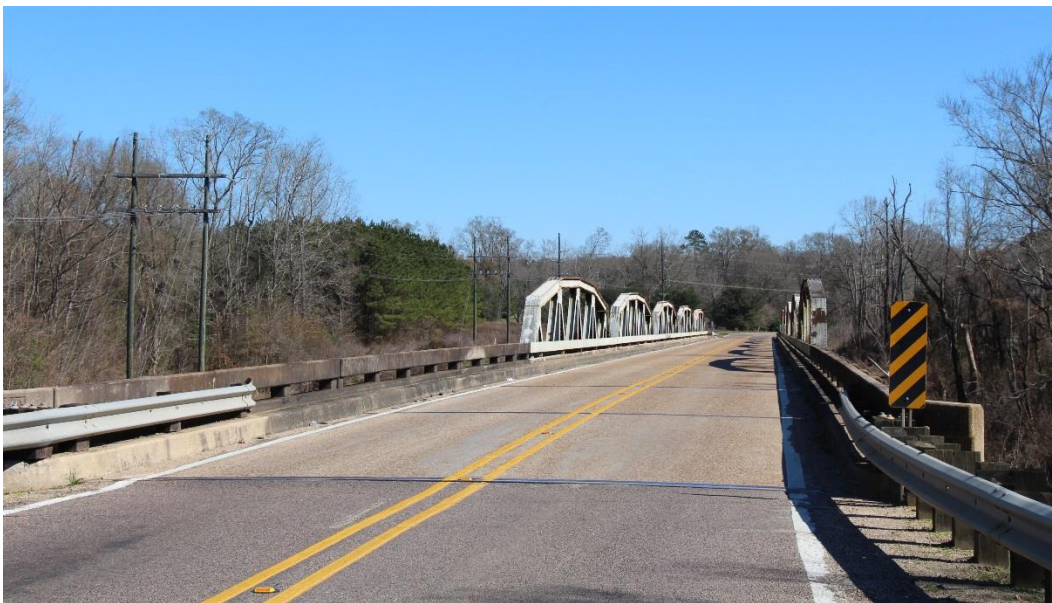
Historic Fabric Photo 1: Steel I-beam approach spans.
