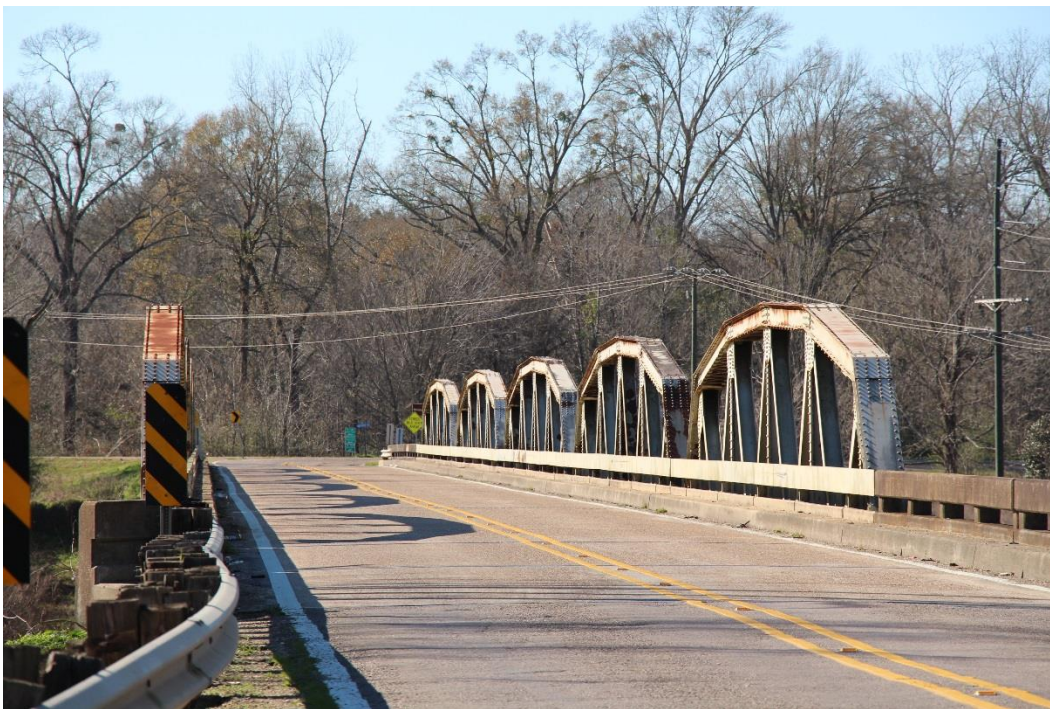
Condition Photo 2: Overview of the truss spans from the top of deck, looking west.
