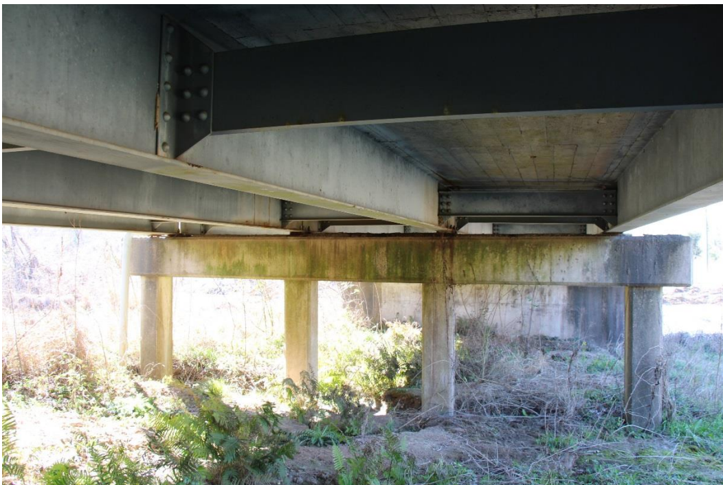
Condition Photo 14: Typical approach span intermediate bent.
